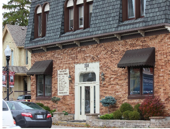
Examples of a non-contributing buildings along Queen Street
