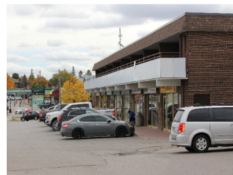
Retail Strip Mall Development with second story residential units along Water Street
