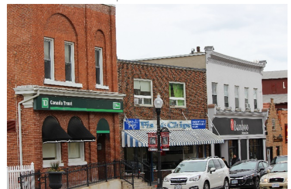
Example of a barrier free access ramp installed at TD Bank on Queen Street.
