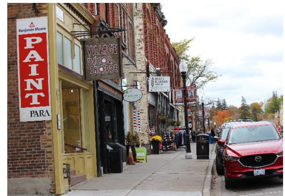
Narrow setbacks and raised entrances on Queen Street can create accessibility issues on can prevent the installation of
