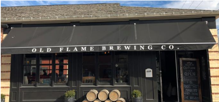
Retractable awning with business name on valance.
